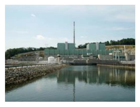
Unit 1 was a 200 MWt, high temperature, gas-cooled reactor that operated from June 1967 to October 1974, when it was permanently shut down. All spent nuclear fuel from Unit 1 was removed from the site, and the Unit 1 spent fuel pool was drained and decontaminated. The Unit 1 reactor vessel, primary system piping, and steam generators remain in place.
