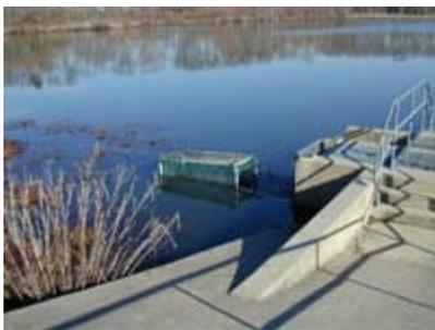
Once fish passage has been provided at a site, biologists [monitor](#) the structure to ensure it is operating properly and that fish are able to ascend above the former blockage. Through biological monitoring, biologists have documented that at least 33 species of fish have ascended a fish passage structure in Maryland, including Maryland's primary target species which are the American shad, hickory shad, alewife and blueback herring.
