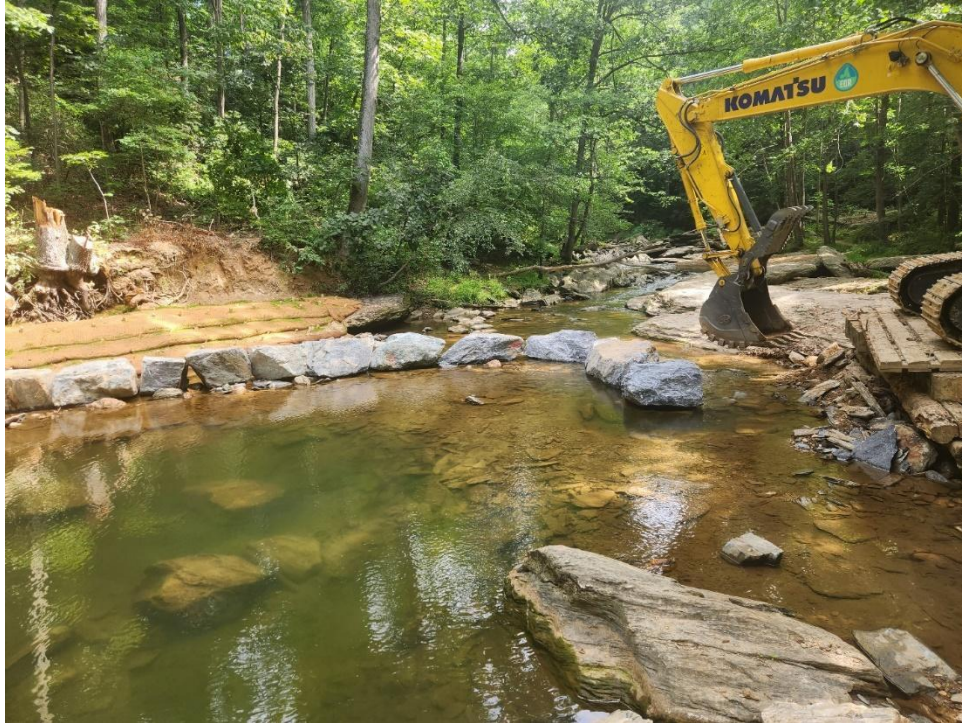
Stream/fish habitat enhancement construction at the Morgan Run Fishing Platform
