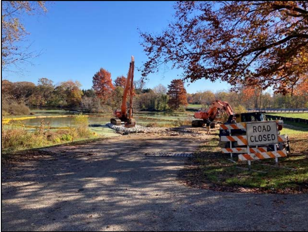
Urieville Lake dredging project
