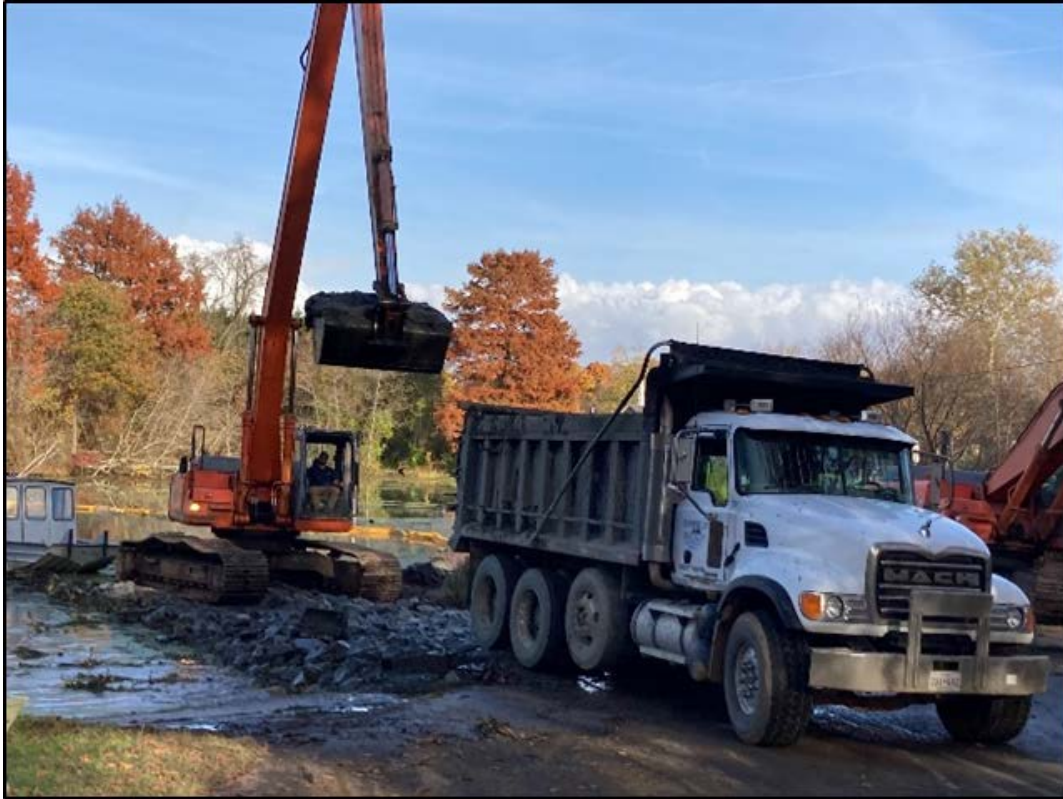
Urieville Lake dredging project
