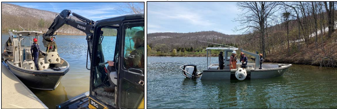
Loading reef balls onto the deployment boat; deploying reef balls
