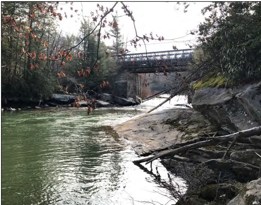
Image 4 – Upstream view of Youghiogheny River taken from the western bank, north of Swallow Falls Road. The bridge to be replaced (Bridge No. G-0020) spanning the river is also shown.
