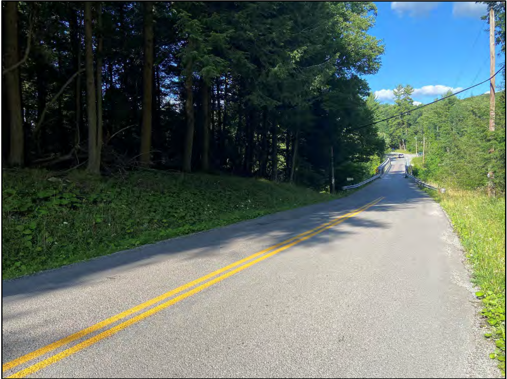
Existing Conditions of the western approach to the Swallow Falls Road Bridge.
