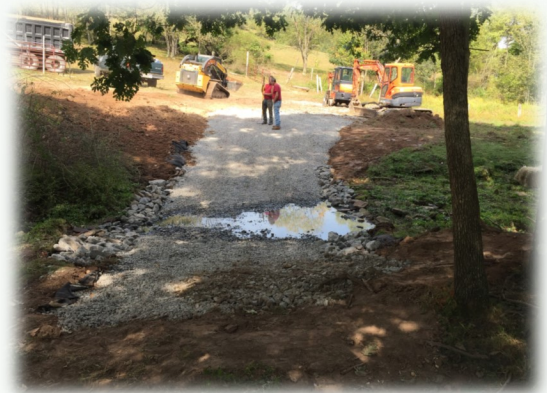
Completed livestock watering area.
